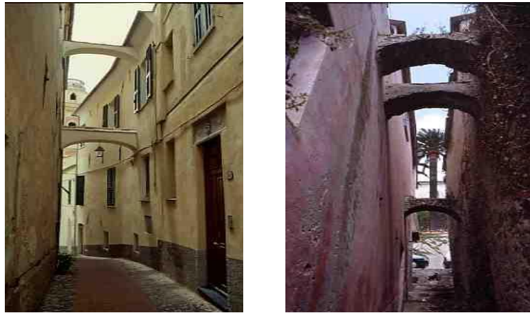
Fig. 7: Examples of arcs of reinforcement in the resort of Diano Castello in Liguria , Italy. (Laurenti, 2002).
