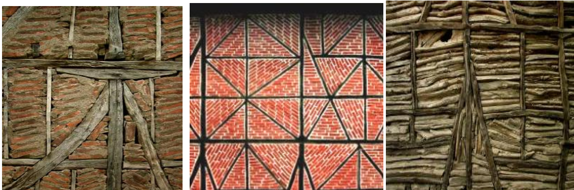
Fig. 4: to the left Hatil, Turkish traditional construction; in the center detail of the variation decorated with construction Himis near Düzce; the right detail of the wall Bagdadi to Golcuk (Gülkan and Langenbach, 2004).
