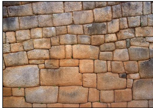
Fig. 9: Detail of a stone wall with close fitting to Machu Picchu.
